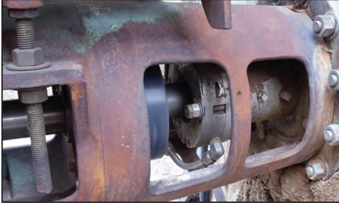
One of two split Inpro/Seal AM Solutions shaft seals installed on white liquor tank agitators.
